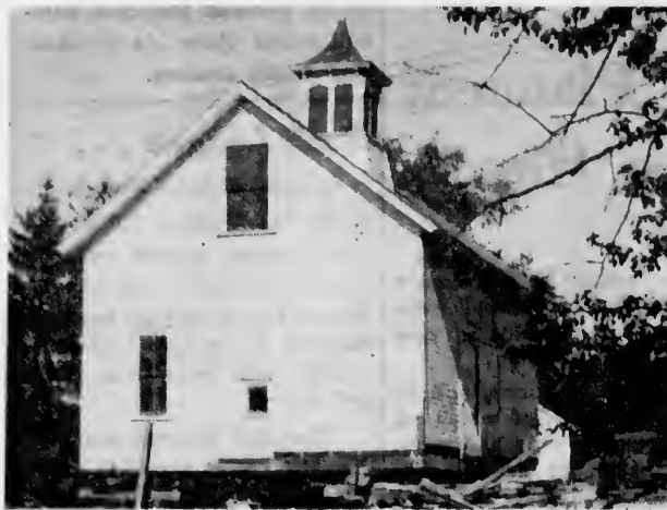
MOVING ON: The old white barn, no longer to house Middlebury's theatre props, is carted out of Voter parking lot forever to make way for the new Language Center.
